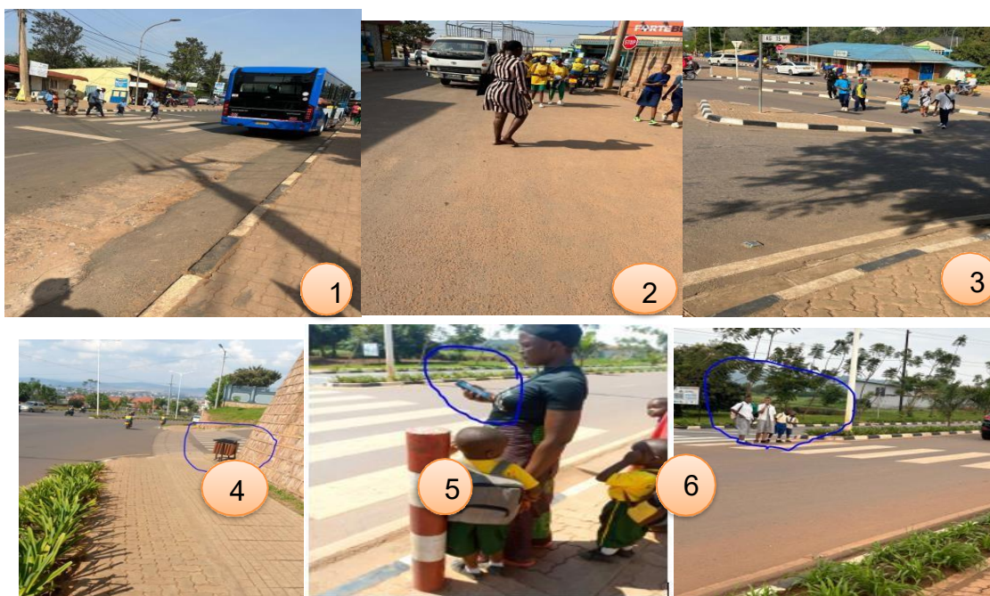
Figure 1: Typical road deficiencies identified
