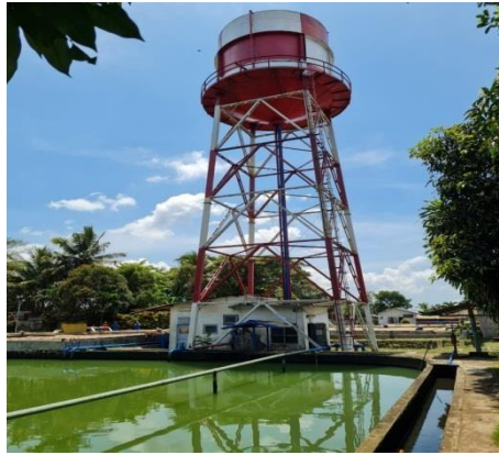
Figure 4. Water Tower' for Production and Hydrant
