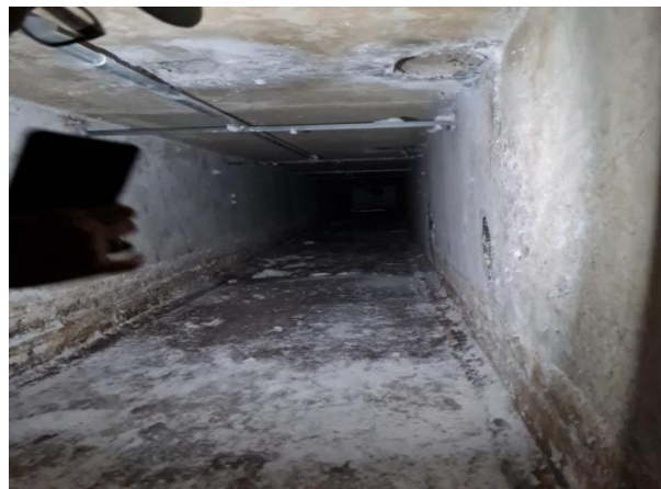
Figure 6. Water Spray Installation' in Underground
