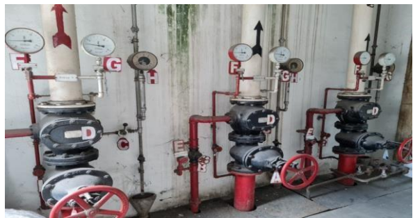
Figure 3. Water Installation' on the Divider to Each Unit
