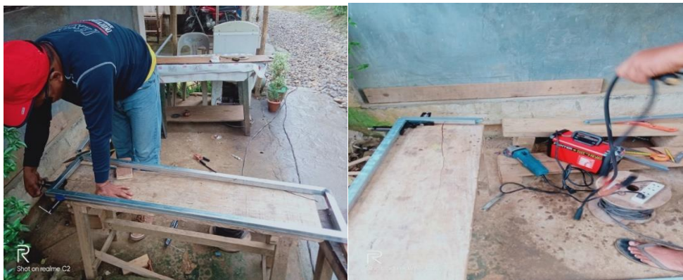
Figure 11. shows the construction of the Vertical Axis Wind Turbine base housing
