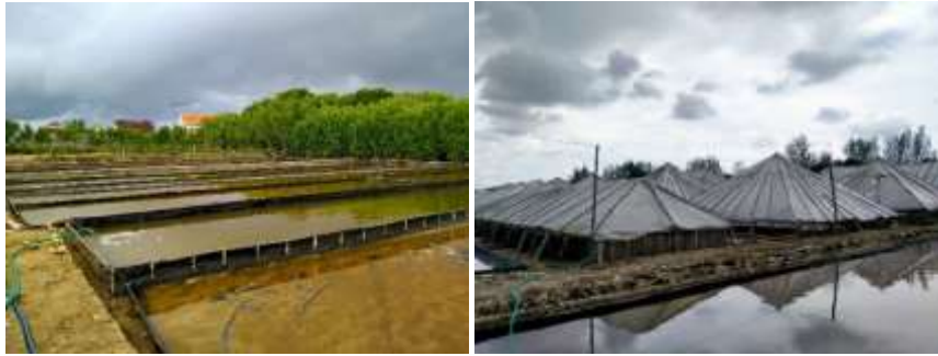
Figure 5. Salt Production with Prism House Technology
