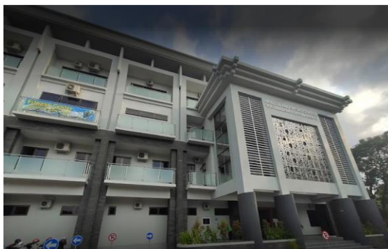
Figure 4. Location of the UNY HSC Fitness Center Building (Source: Personal Documentation)
