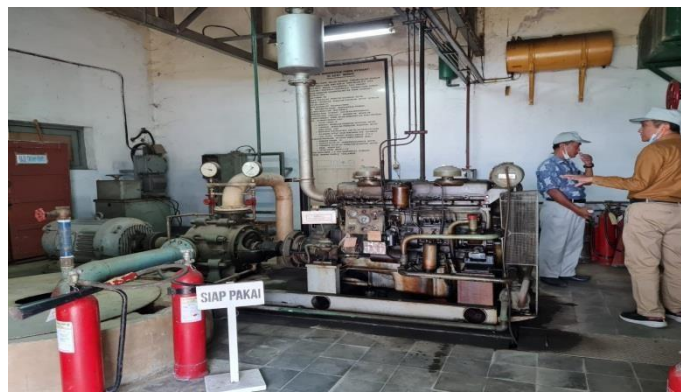
Figure 5. Hydrant Pump
