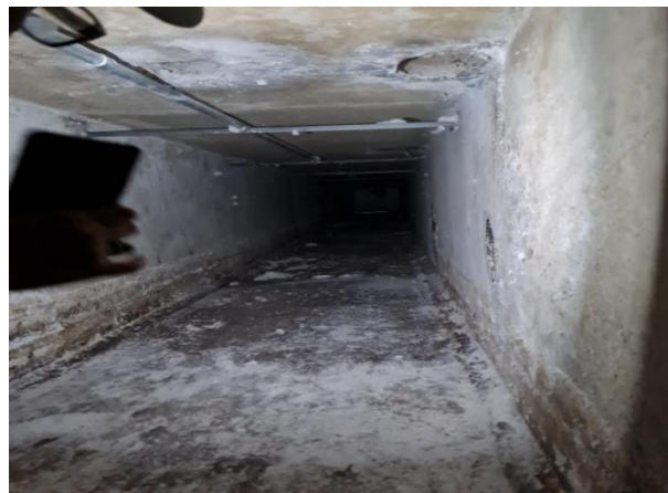
Figure 6. Water Spray Installation' in Underground
