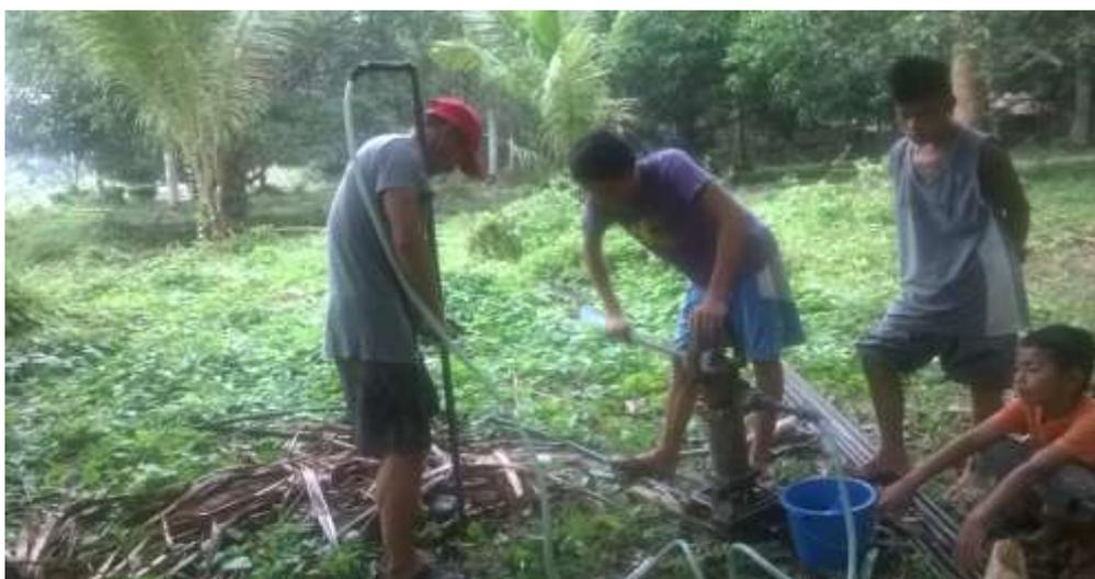
Figure 3. Local drillers using locally fabricated drilling rig during the actual manual drilling for well logging in the study area
